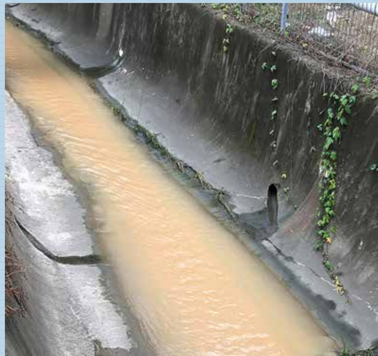
Above: Sediment laden water from construction site at Harris Park; Right: Residential development at Wentworth Point on the Parramatta River.
