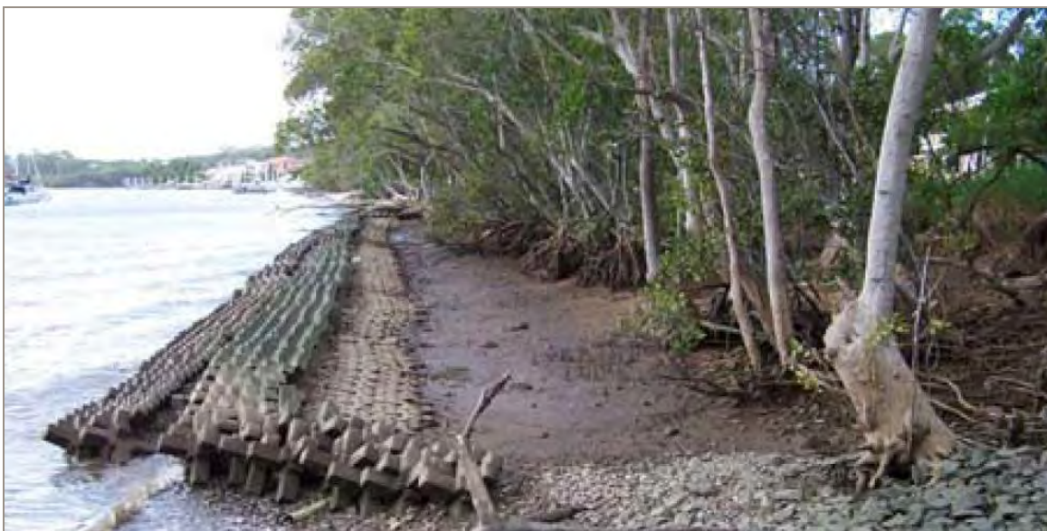
Figure 5-11. A-Jack units installed in front of mangroves at Charles Holm Park on the Coomera River QLD (Derbyshire 2006)
