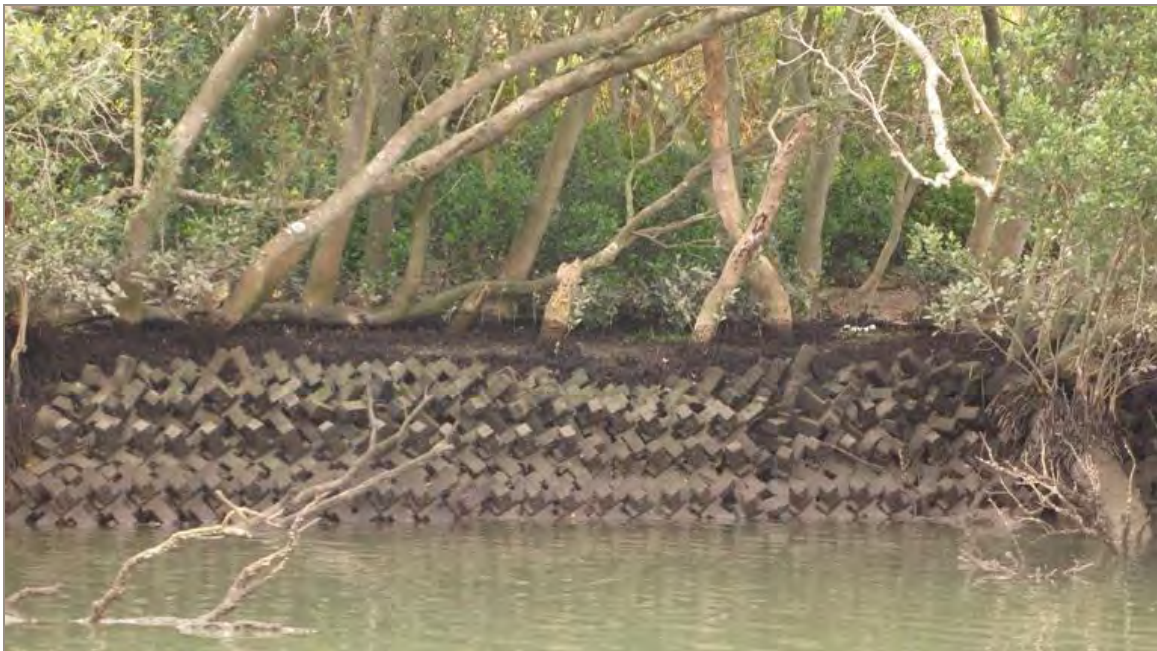
Figure 5-10. A-Jack units installed in front of mangroves on the Parramatta River upstream of Silverwater Bridge
