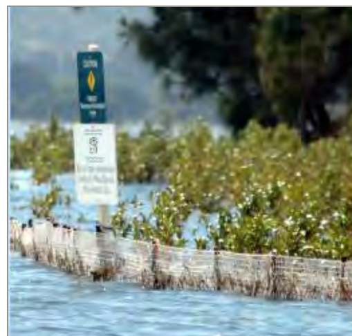
Figure 5-18. (a) Coir logs installed on the banks of the Lower Murray River and (b) Tidal riverbank restoration using mangroves (Southern Rivers CMA)
