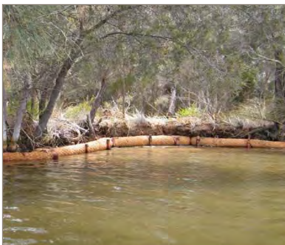
Figure 5-18. (a) Coir logs installed on the banks of the Lower Murray River and (b) Tidal riverbank restoration using mangroves (Southern Rivers CMA)
