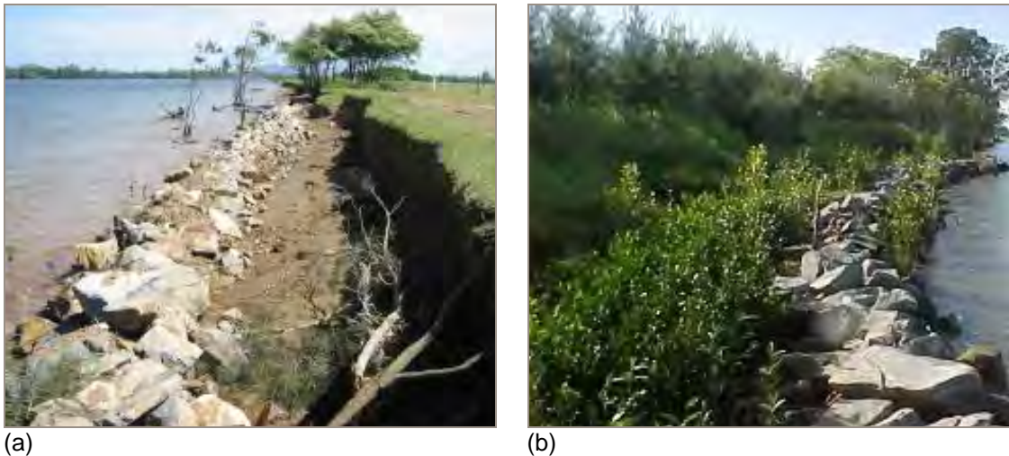
Figure 5-15. Rock fillet work allowing mangrove seedlings to regenerate, (a) Hastings River (b) Dumaresq Island, Manning River
