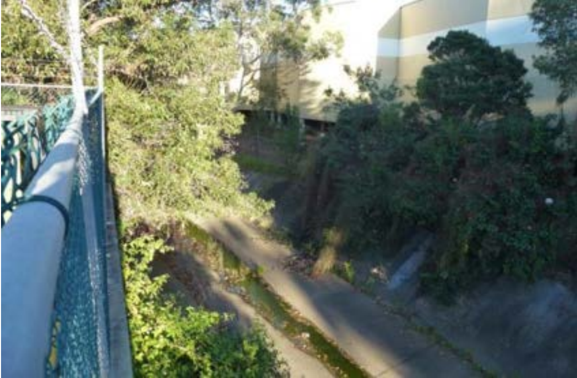
Figure 77 Corridor from Foundry Road
