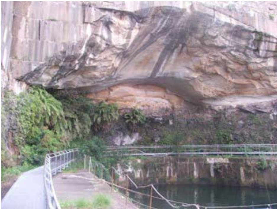
Figure 72 Woolwich dock walkway
