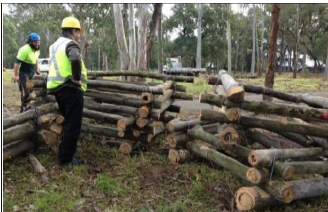
Figure 30: Construction of fish crates before being submerged into low velocity water body (GSLLS 2015).
